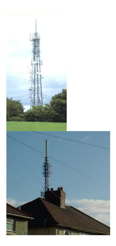
Each base station provides coverage over a limited area, or cell, in the area around the site. That's why in some countries mobile phones are called cell phones. To offer comprehensive network coverage, the cells must overlap each other like a patchwork quilt, so that users can move from one cell to another without breaking connection. As each cell can only handle a limited
